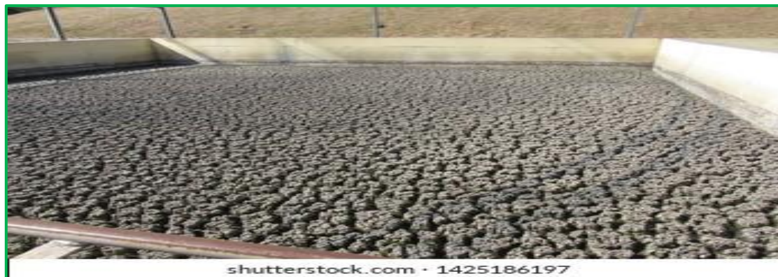
Figure: 1 Sewage sludge in outlet tank produced
