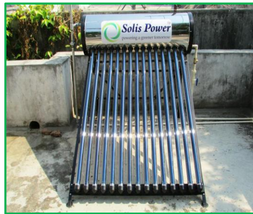
(Solar water heater)
