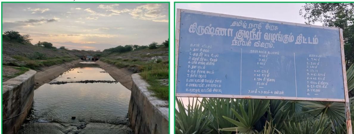
Zero point uthukottai, bridge, pedukuppam, Andhra Pradesh- 602026
